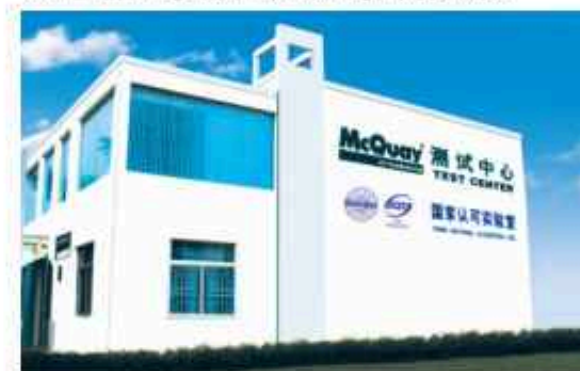
This test room is Nationally Recognized Testing Laboratory
